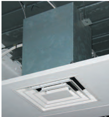
Typical Installation with Side Entry Plenum
